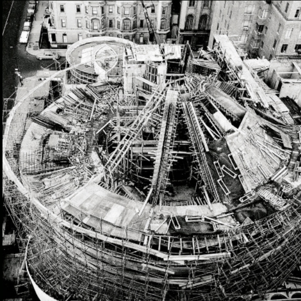
Construction of the main rotunda, ca. 1958. Photograph by William H. Short © The Solomon R. Guggenheim Foundation, New York.
